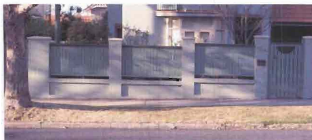
Sympathetic fence with masonry base, timber picket panels and emphasised masonry plers. Wider spacing of the pickets would increase the sympathetic character of the fence
