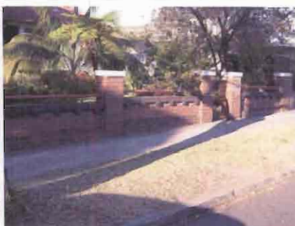
Original Federation fence of two tone face brick with pipe rails
