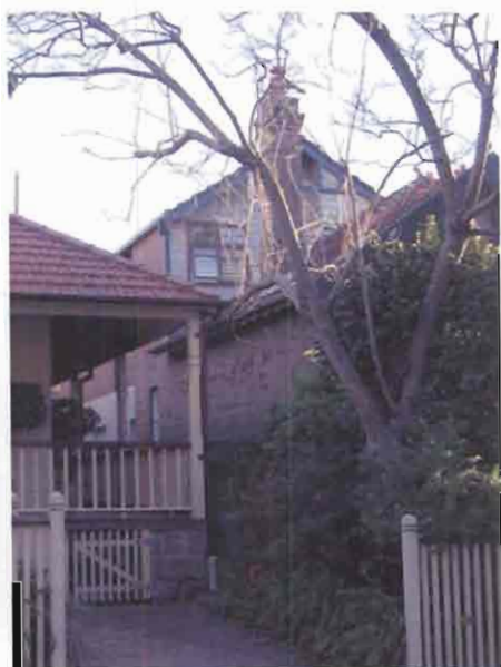
Another example of a sympathetic rear addition which is setback from the façade, retains the main section of the dwelling and does not impact on the streetscape
