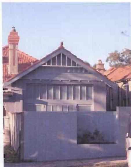
Intrusive Alterations - Façade Detailing has removed original character
