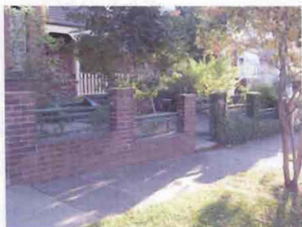
Original Federation period fence with face brick, pipe rails and iron mesh panels
