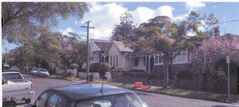
Row of typical Federation period detached and semi-detached dwelling along the northern side of Glover Street (1 & 2 Contributory)
