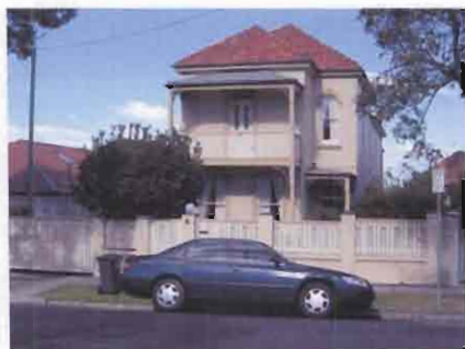
Only two storey Federation period dwelling in the street (2 Contributory)
