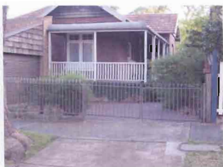
Intrusive powder coated pool-type fencing
