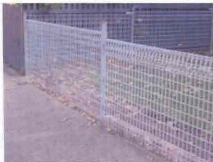
Intrusive Fence of Welded Steel Mesh
