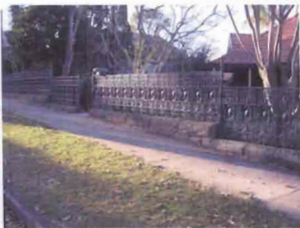
Original and significant Federation period cast iron panel fence on sandstone base
