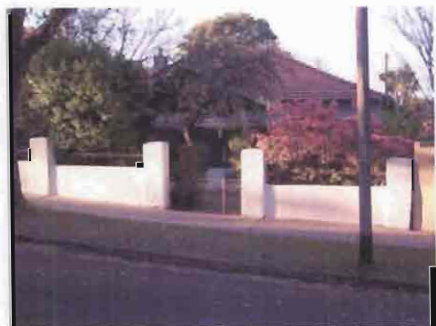
Original inter war fence roughcast render base and pipe rails
