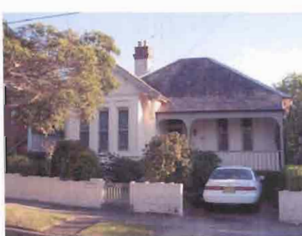
The Intrusive treatment of the façade by the painting of the face brick
