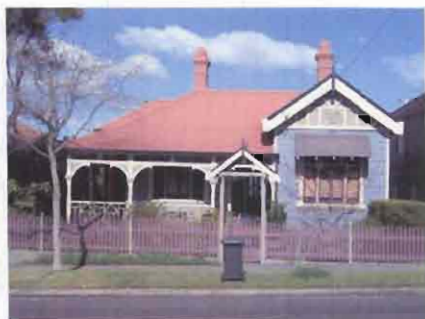
Heritage Item at No 48: Double fronted timber board cottage
