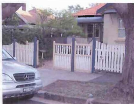
Sympathetic Federation style timber picket fence and gate for car space
